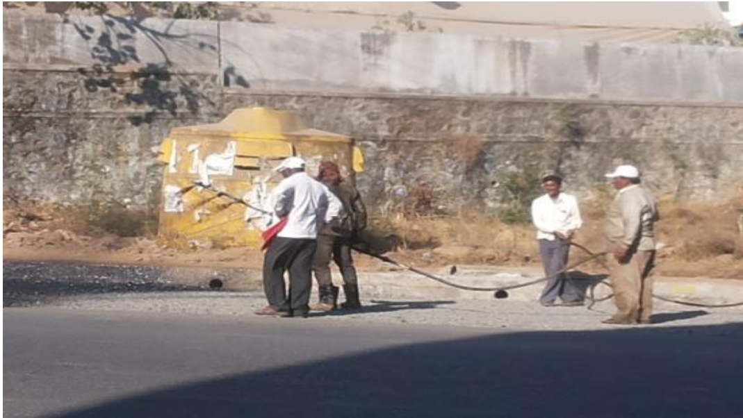
Fig.6 Intelligent Sprayer (Actual photograph at site)
